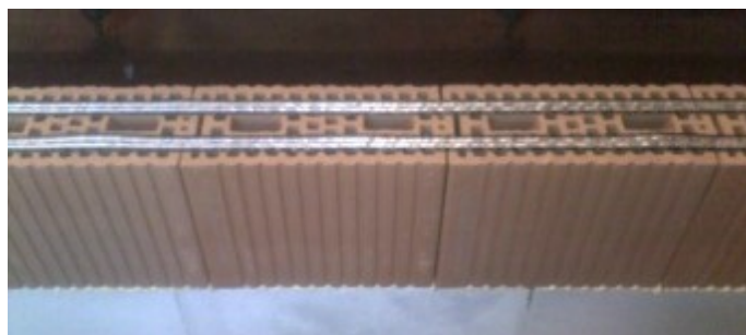
Figure 16 – Armature de joint horizontal
